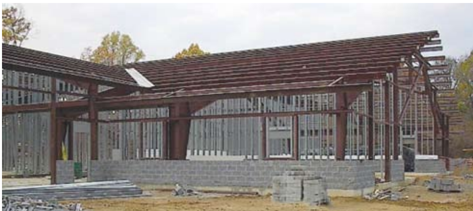
Foxcroft School maintenance building in Middleburg
