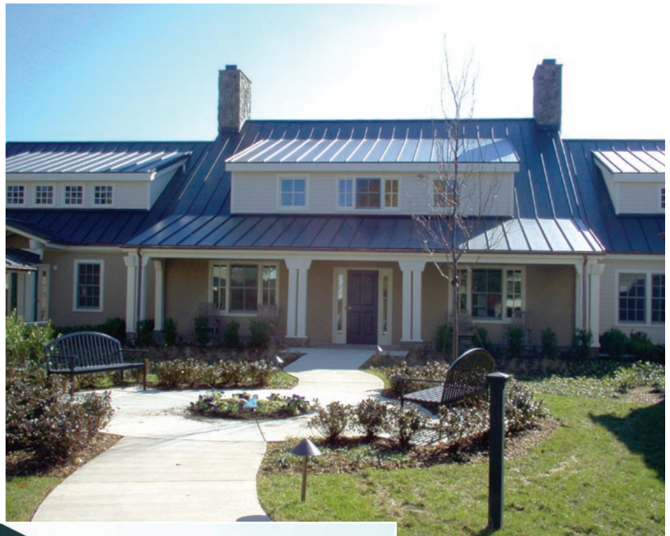
The Courtyard at Middleburg Office Building with parking below
