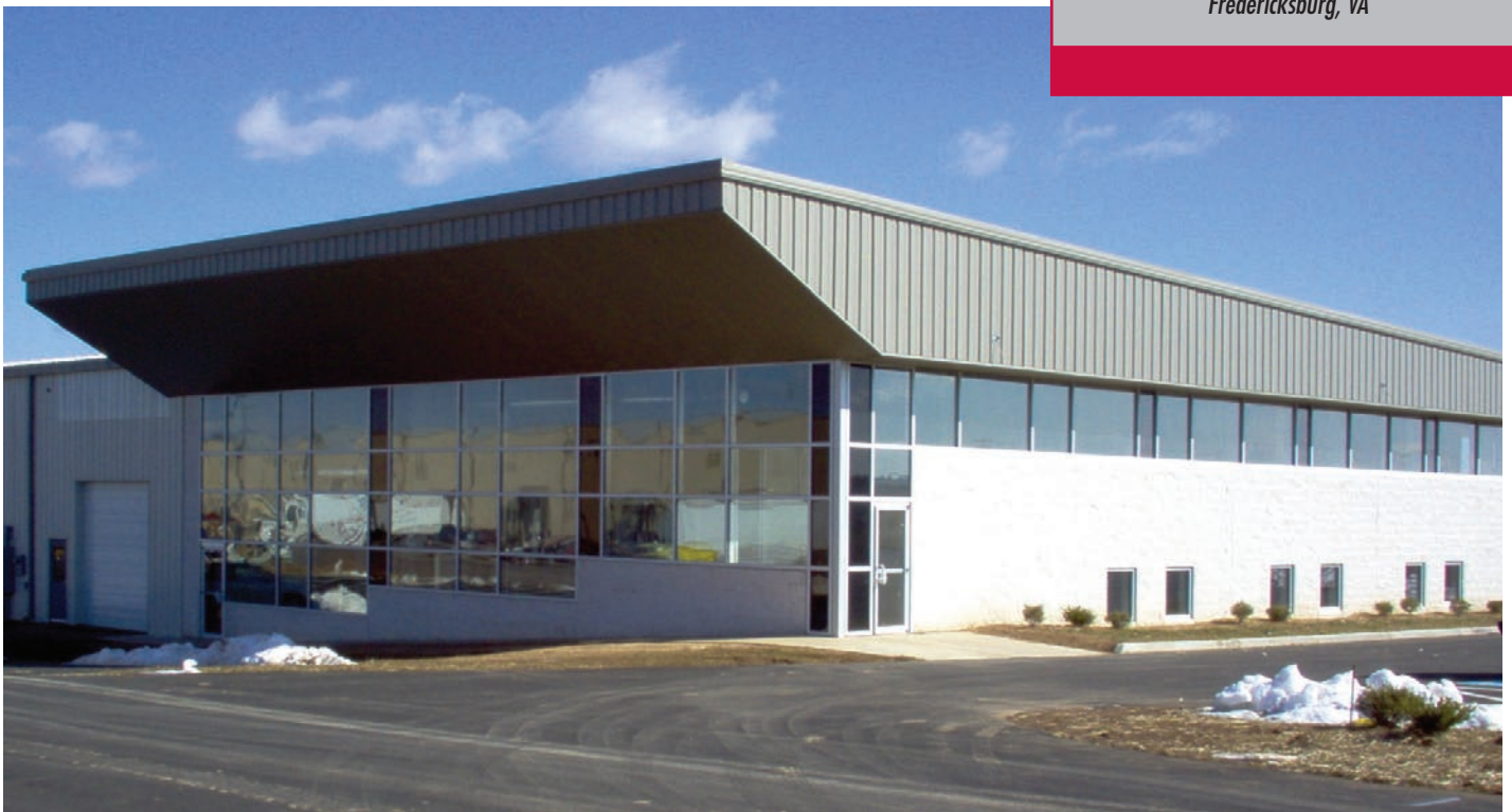
American Manufacturing's new Culpeper facility.
