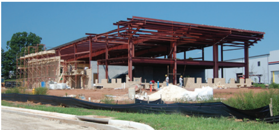
The Morais Investment building in Manassas, currently under construction
